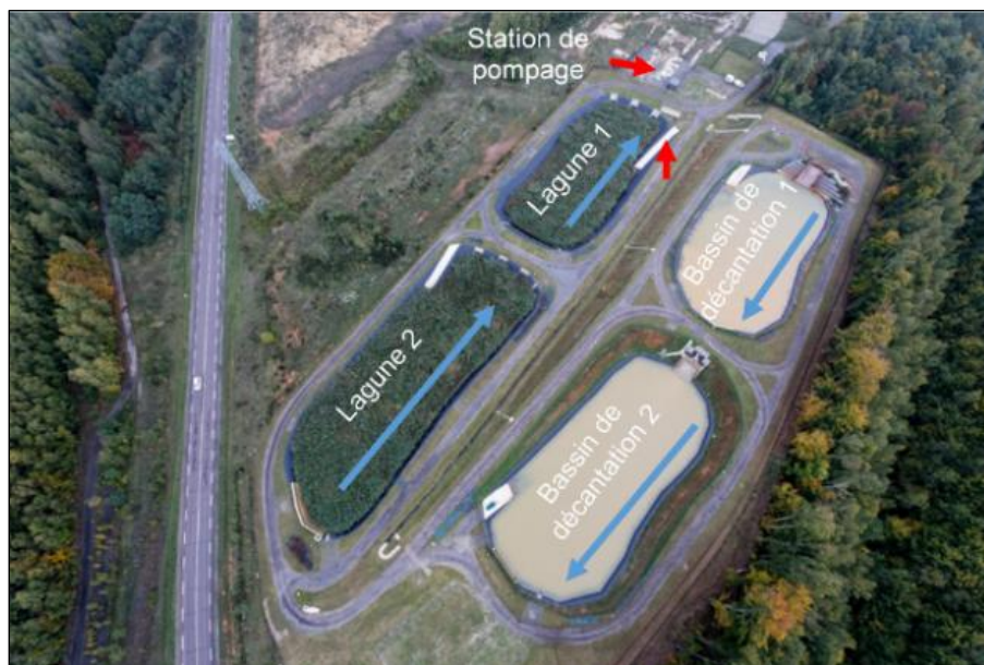
Figure 4 : Water pumping and treatment station in the Lorraine coal basin (source: BRGM/DPSM)
