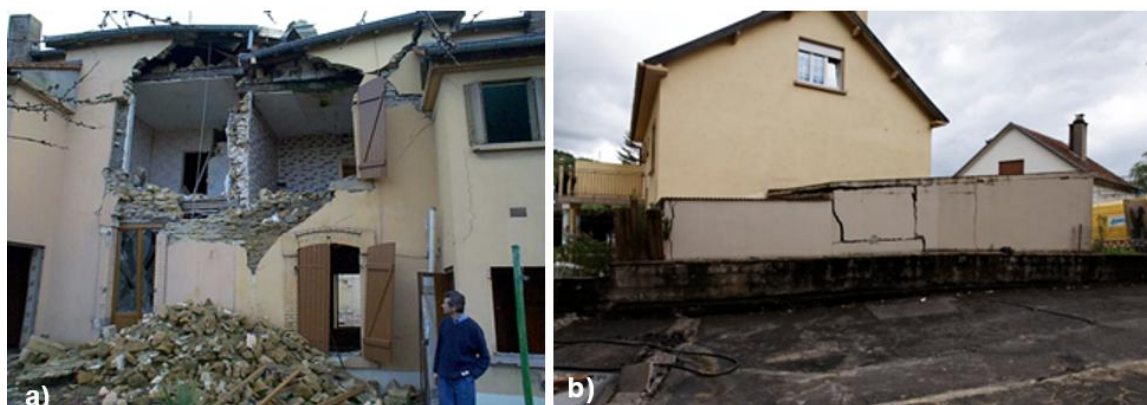
Figure 2 : (a) Damage caused by subsidence in Auboué (1996), (b) Collapse in Moyeuve (2012)
