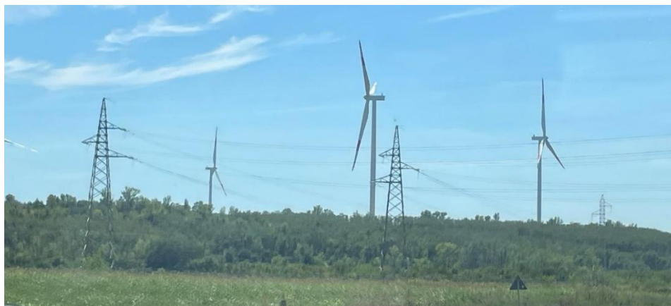
Figure 5: Constructed wind park on the external dump
