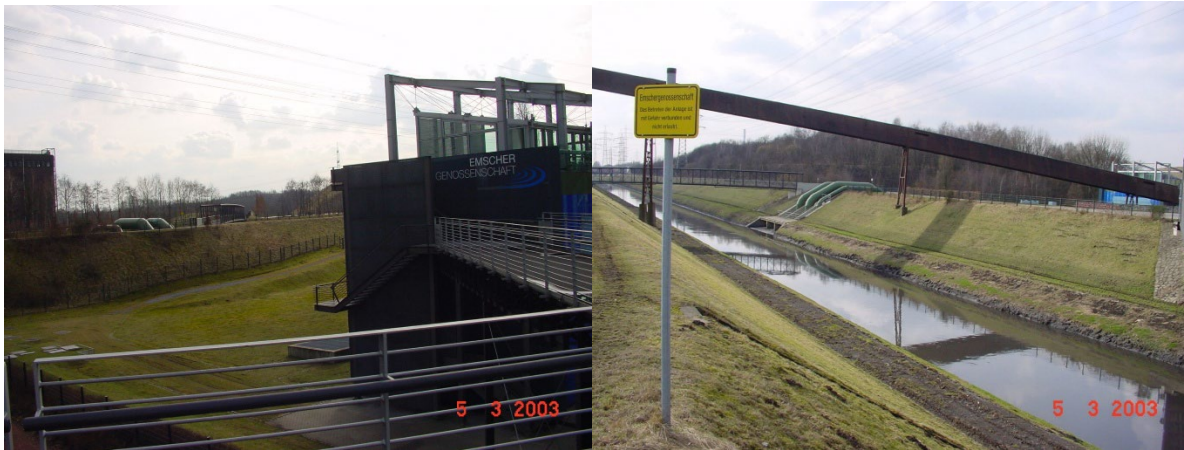
Fig. 27: In Ruhr Area exist about 160 pumping stations like in the picture. Without pumping the water table will rise up to 7 meters above the dyke (own picture).
