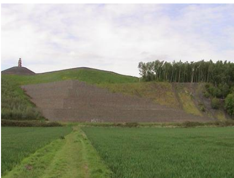
Fig. 17 and 18: Covering dump Rheinelbe with soil and gabion wall (own pictures)
